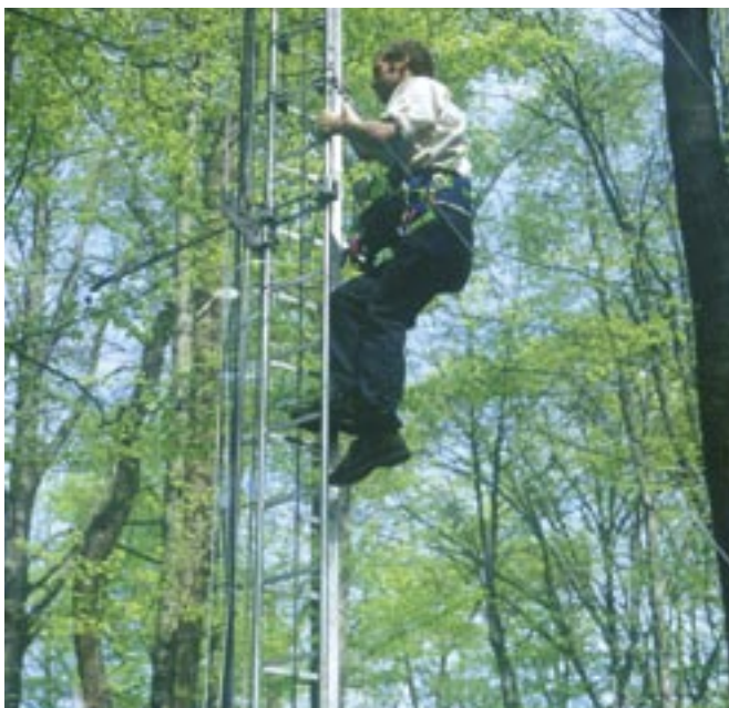
Maintenance work in micrometeorological tower – Hainich national park, Germany.
